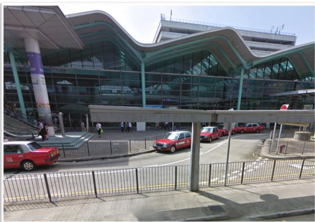
Outside Hung Hom MTR Station, Exit C
